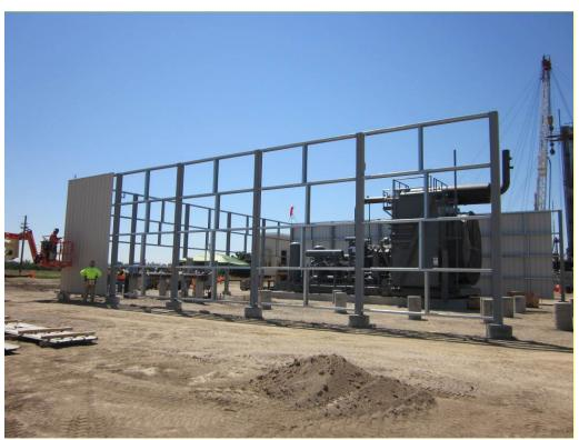
Photo 2: Soundwall work at temporary compressor placed at the remote well pad site.
